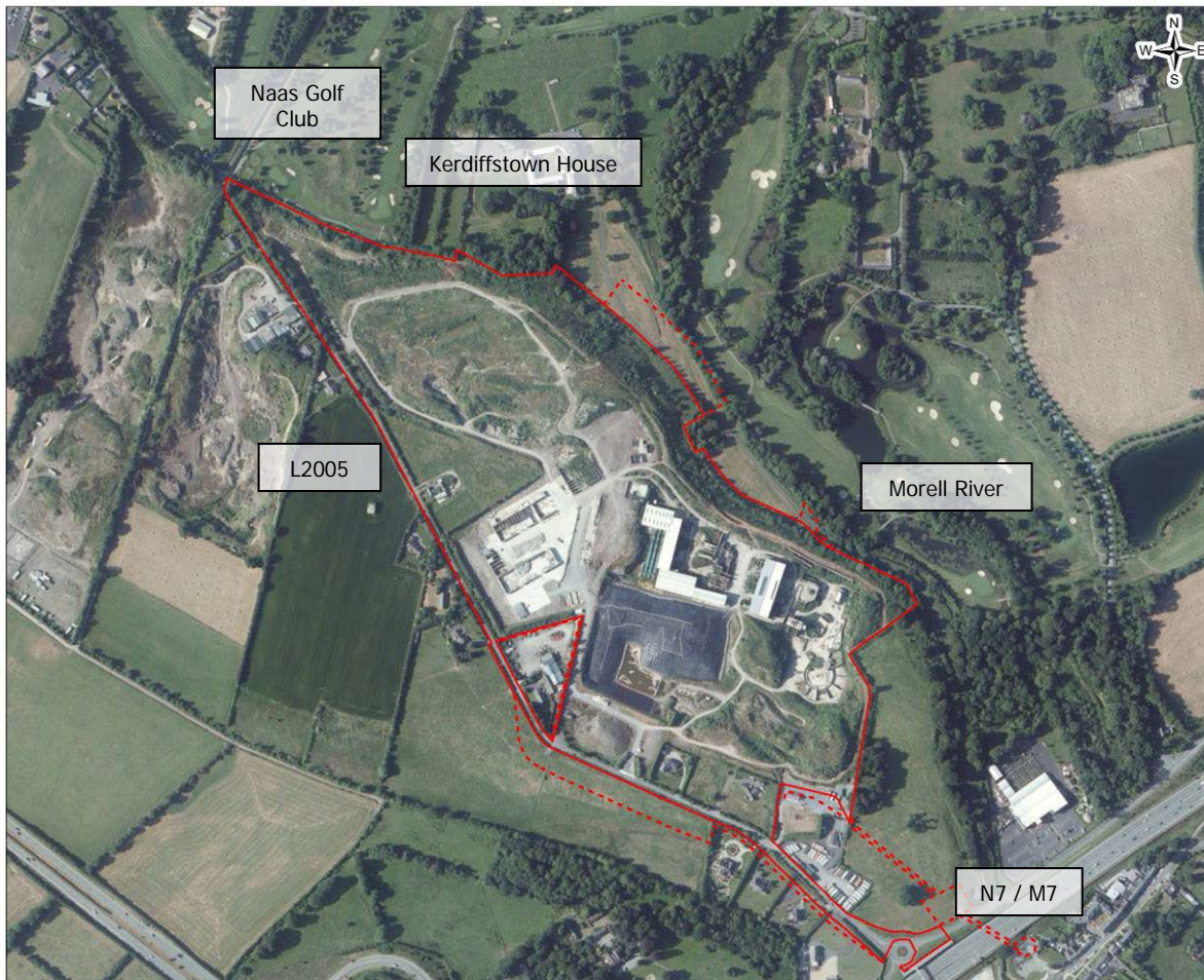
Figure 2.2 Aerial view of the site (indicated in red) and proximate land uses
